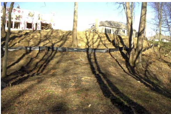
Silt fence installed to protect Swan Creek.
