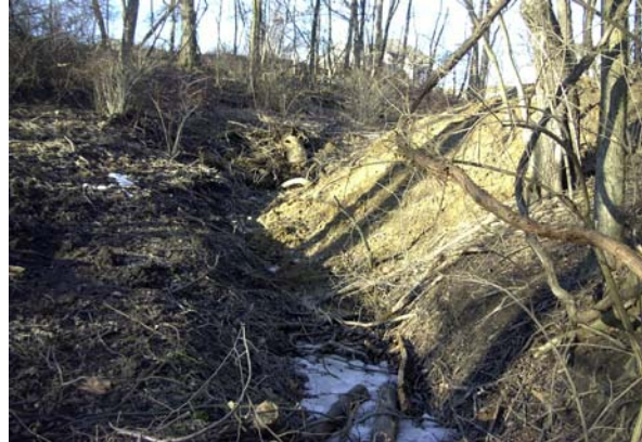
Fill placed in a natural drainage channel.
